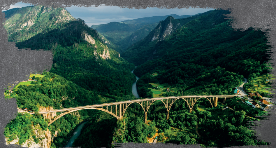
Aerial View of Durdevica Tara Arc Bridge in the Mountains, Foto: ronedy, Fotolia
